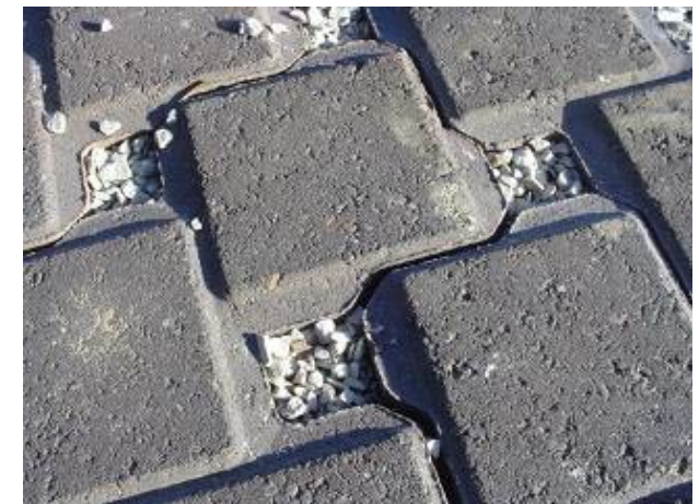
Porous parking lot materials incorporated as part of the overall parking lot plan allow storm water to be absorbed gradually (4)
