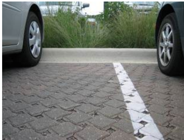
Porous parking lot materials incorporated as part of the overall parking lot plan allow storm water to be absorbed gradually (4)
