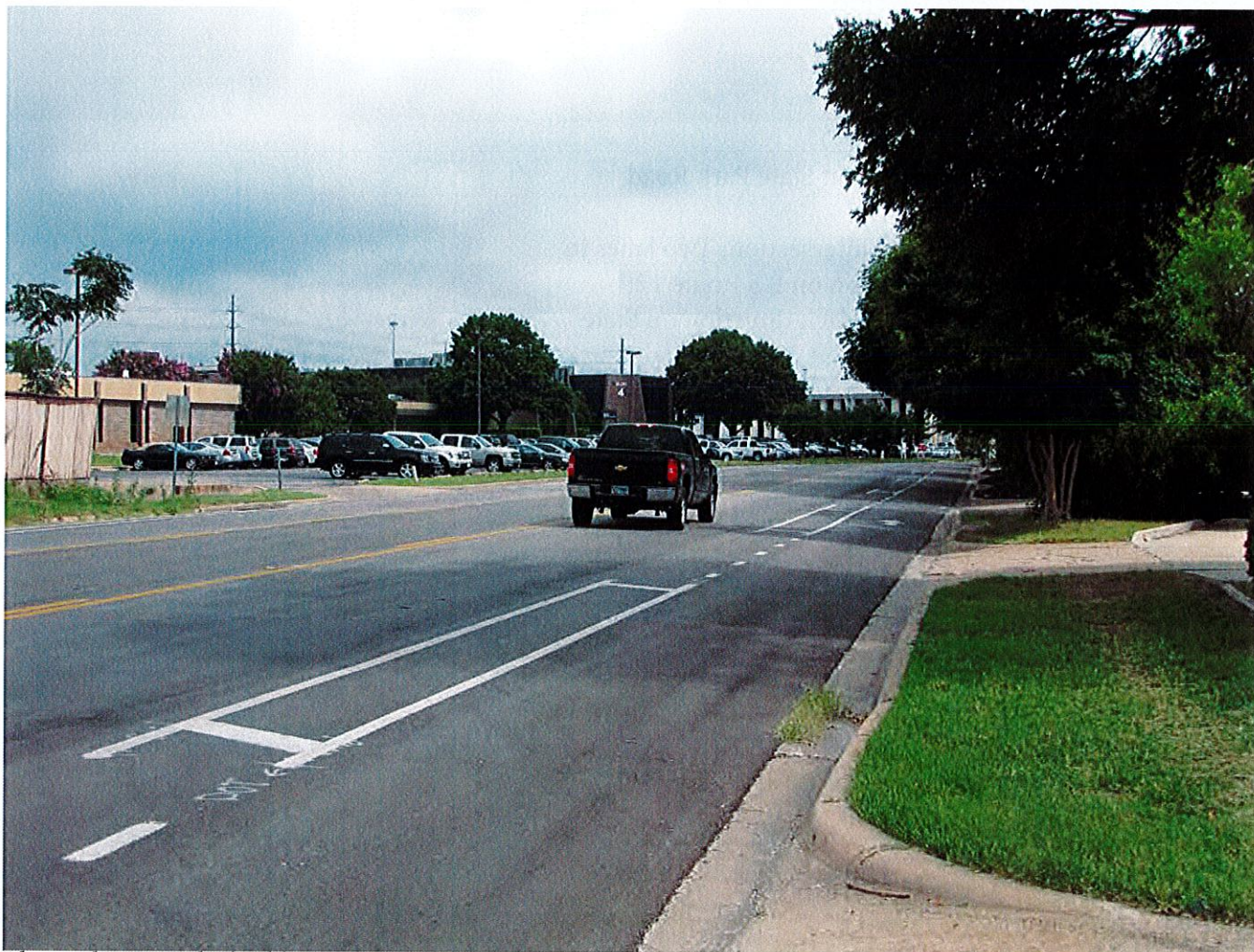
Photo showing dashed line treatment at street and driveway crossings (Source: Bikevote.org)
