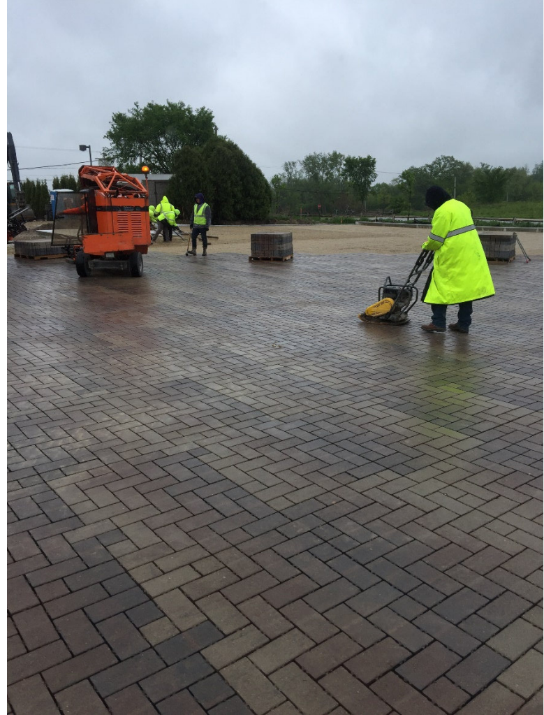
Permeable pavers installation
