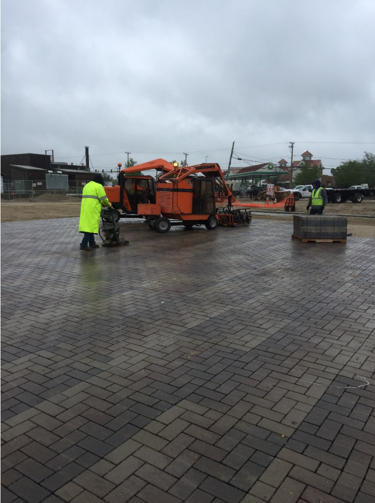
Permeable pavers installation
